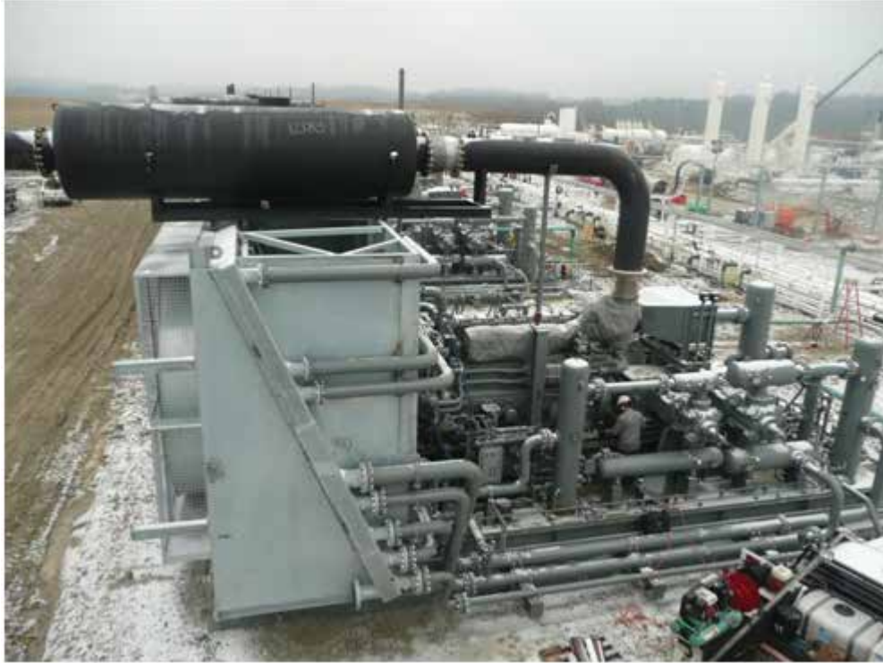
Figure 3.5 — Gas compressor package with vertical air cooler. For a size reference, note the service technician directly beneath the exhaust stack at engine rear.
